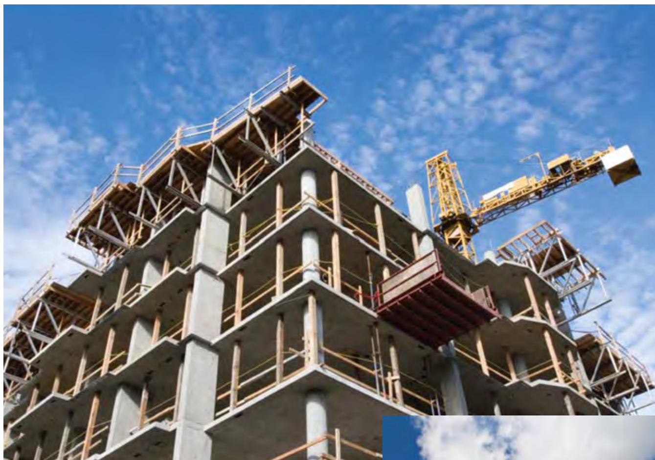
Construction Elevator Emergency Stops
