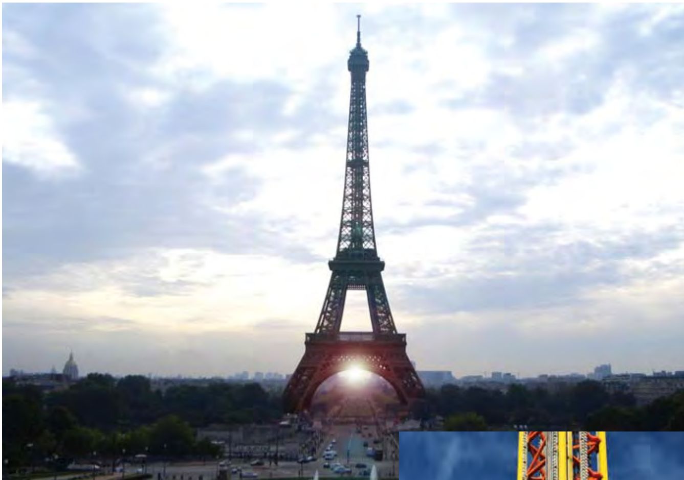
High Speed Elevator Applications
