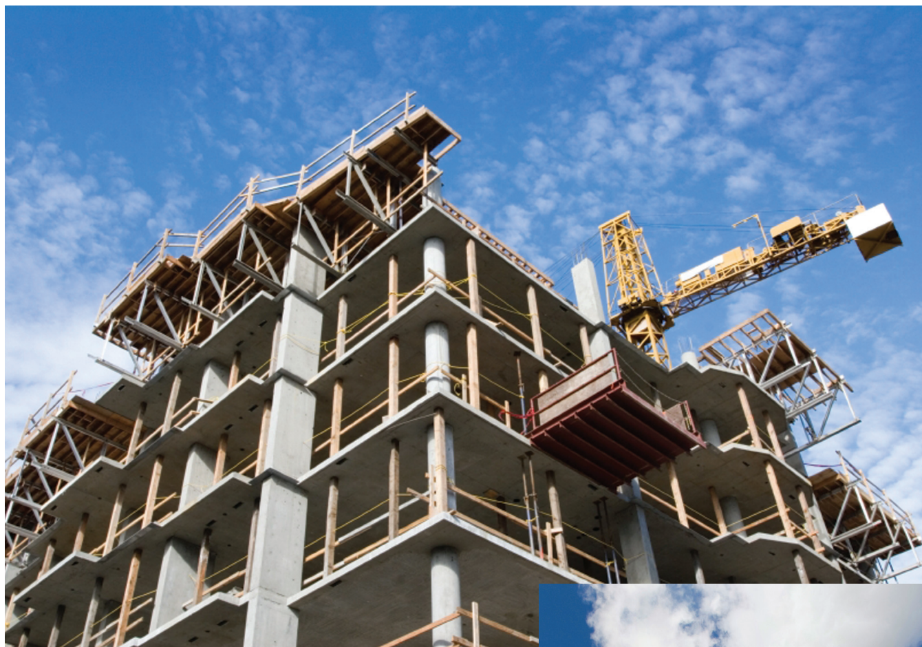
Construction Elevator Emergency Stops
